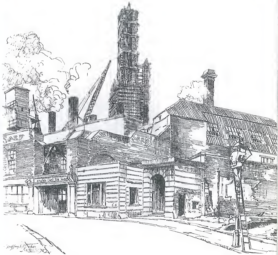
Bankside Power Station under construction. A view of 1952 from Skin Market Place, off New Globe Walk. A pen and ink drawing by Geoffrey Fletcher.
